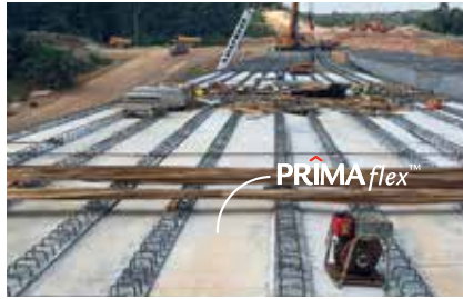
PRIMAflex™ boards are ready for concrete pouring without need for additional support.
